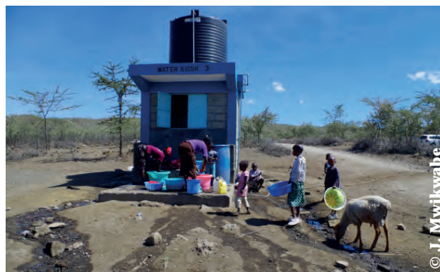
Water point at RAPland, Kenya.
